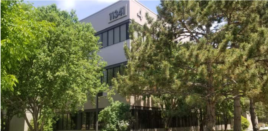
Building 4 - Department of Finance, Licensing
