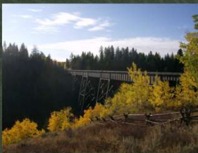
A trestle on the Ashton-Tetonia trail
